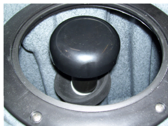
Float Shutoff Assembly
