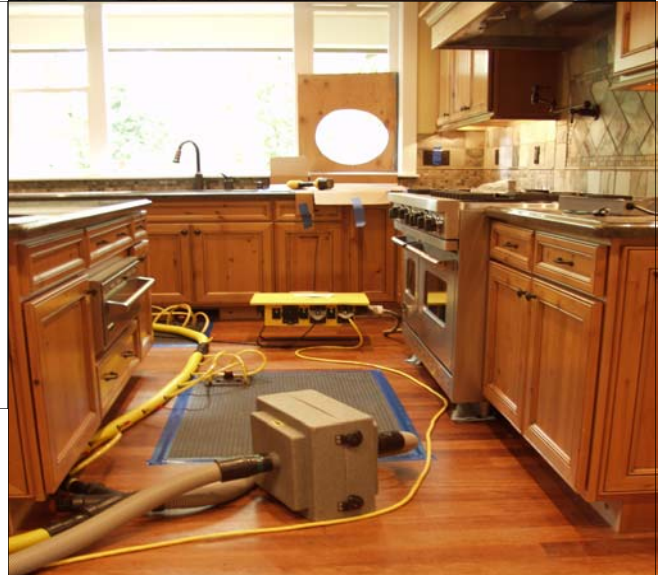
DURING Combination of 8 Point (which were modified by cutting between the grid sections) & Multi-Port Panels
