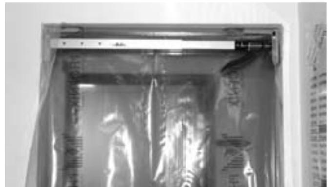
Figure 3: Properly installed Phoenix Quick chamber
