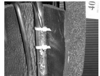
**Figure 4: Thermistor attached to the refrigerant line.**
